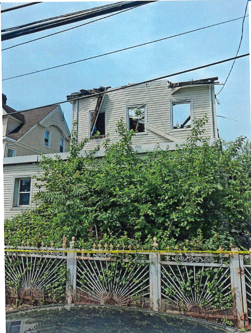
Photo 2 — Street-level view showing perimeter fencing, vehicle in yard, and MVDPW barricade
