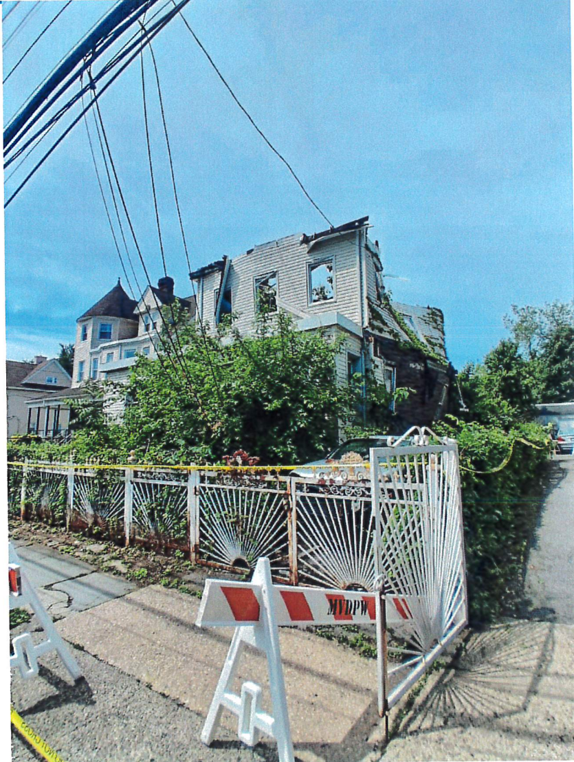
Photo 1 — Front elevation view of structure
