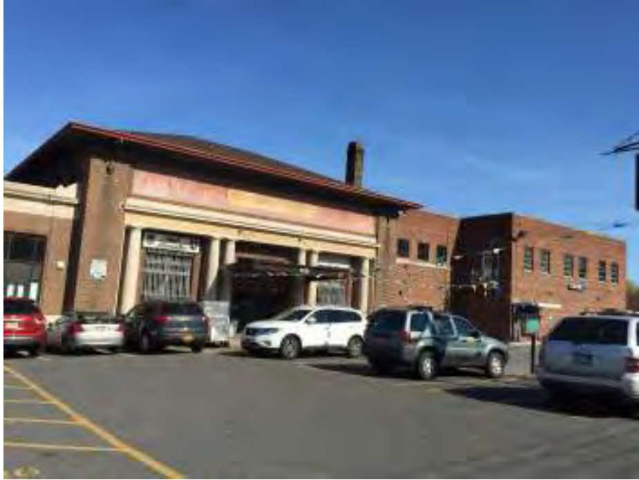
Photo 1: General view of the Site.
