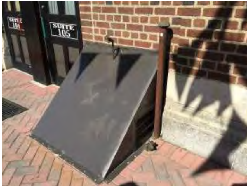
Photo 10: Fill port for the AST located in the east of the building.
