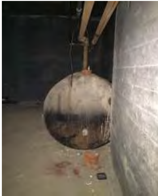
Photo 10: A 1,000 gallon Above-ground Storage Tank (AST) located in the basement.
