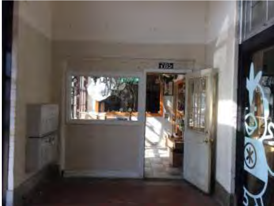
Photo 6: Interior view of the Building
