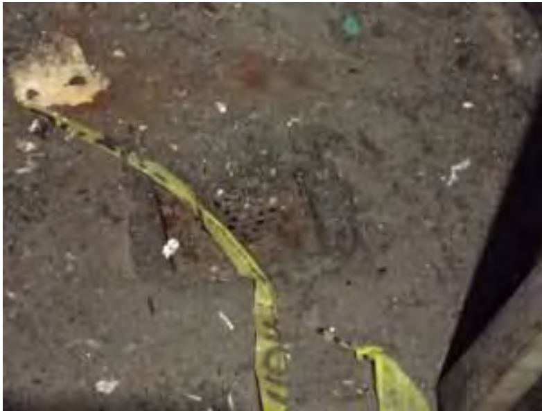
Photo 10: Floor drain located in the basement.
