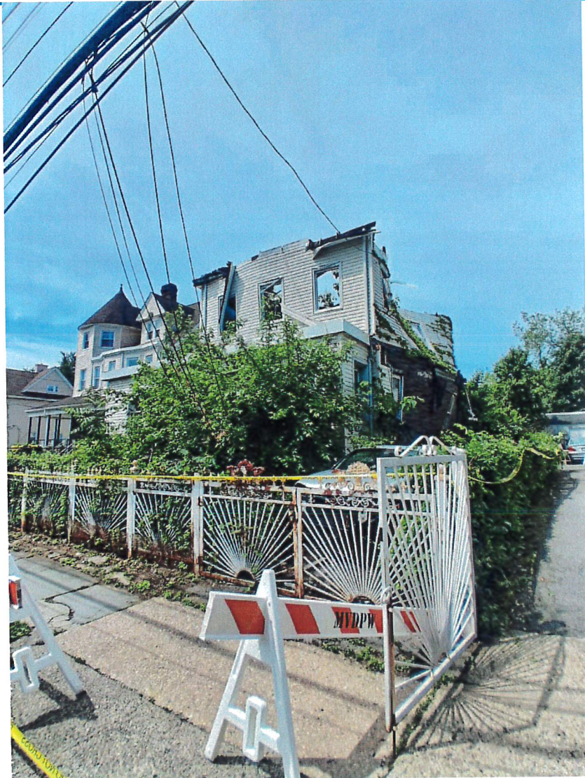
Photo 1 — Front elevation view of structure
